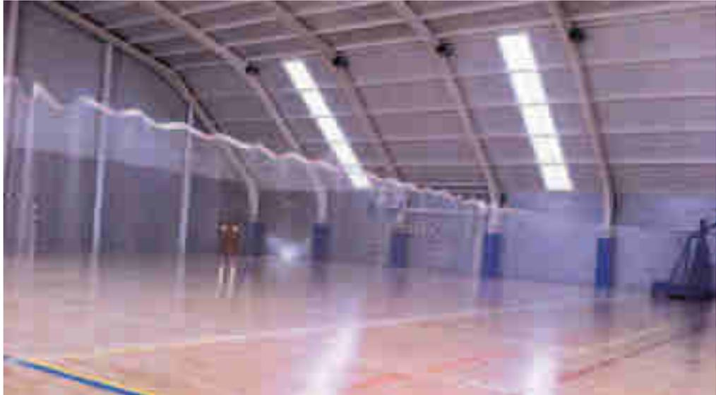
Manually operated curtain with a sideways movement. The system is set up on a tripod at one of the ends from which a cable provides anchoring to the wall the curtain runs along. For use when anchoring to a structure is not possible, or alternative solutions are very costly.
